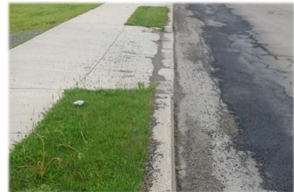
Main Street: Potholes and loose gravel – bad for cyclists!
